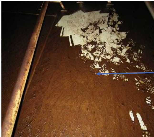
Microbial biofilm in jet fuel storage tank
