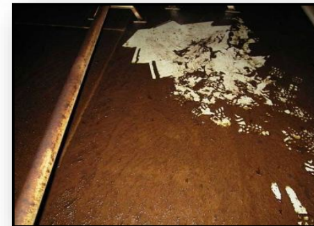
Supply & Distribution tanks
