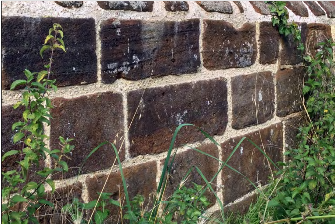
C.08: GOOD QUALITY REPOINTING OF A SQUARED RUBBLE WALL
